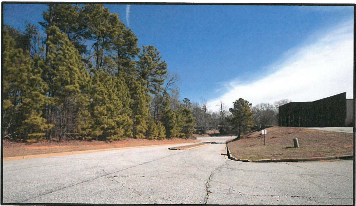
Photo 2—Looking east on Camelot Court towards Camelot Drive.
