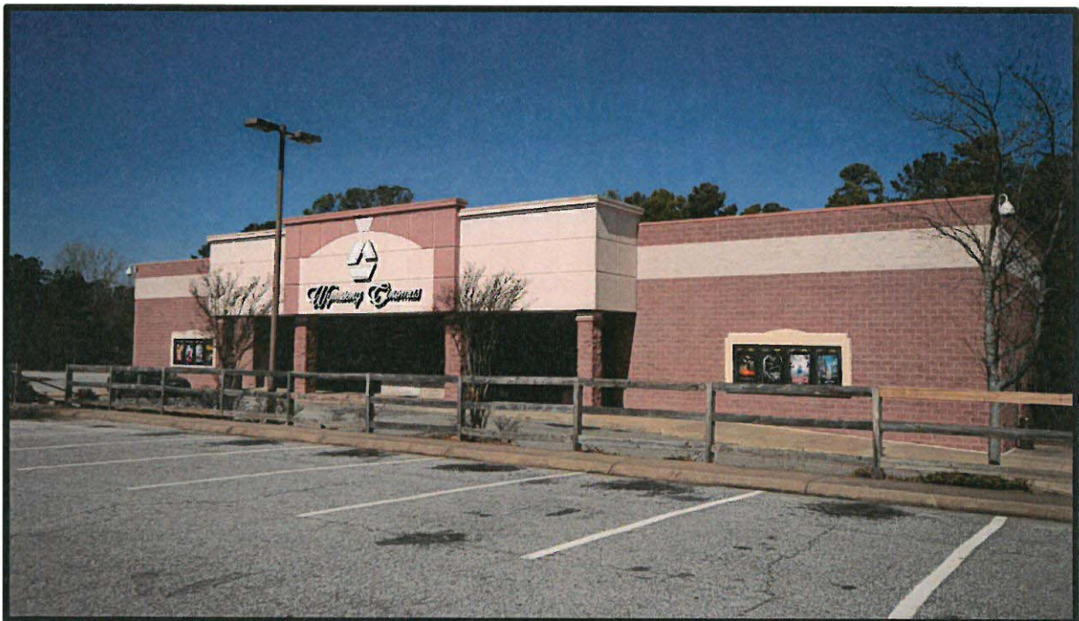
Photo 6—The movie theater that is adjacent to the site.
