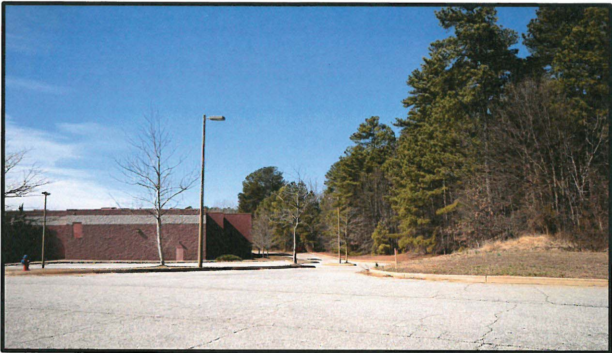
Photo 5—Looking northwest towards the site.
